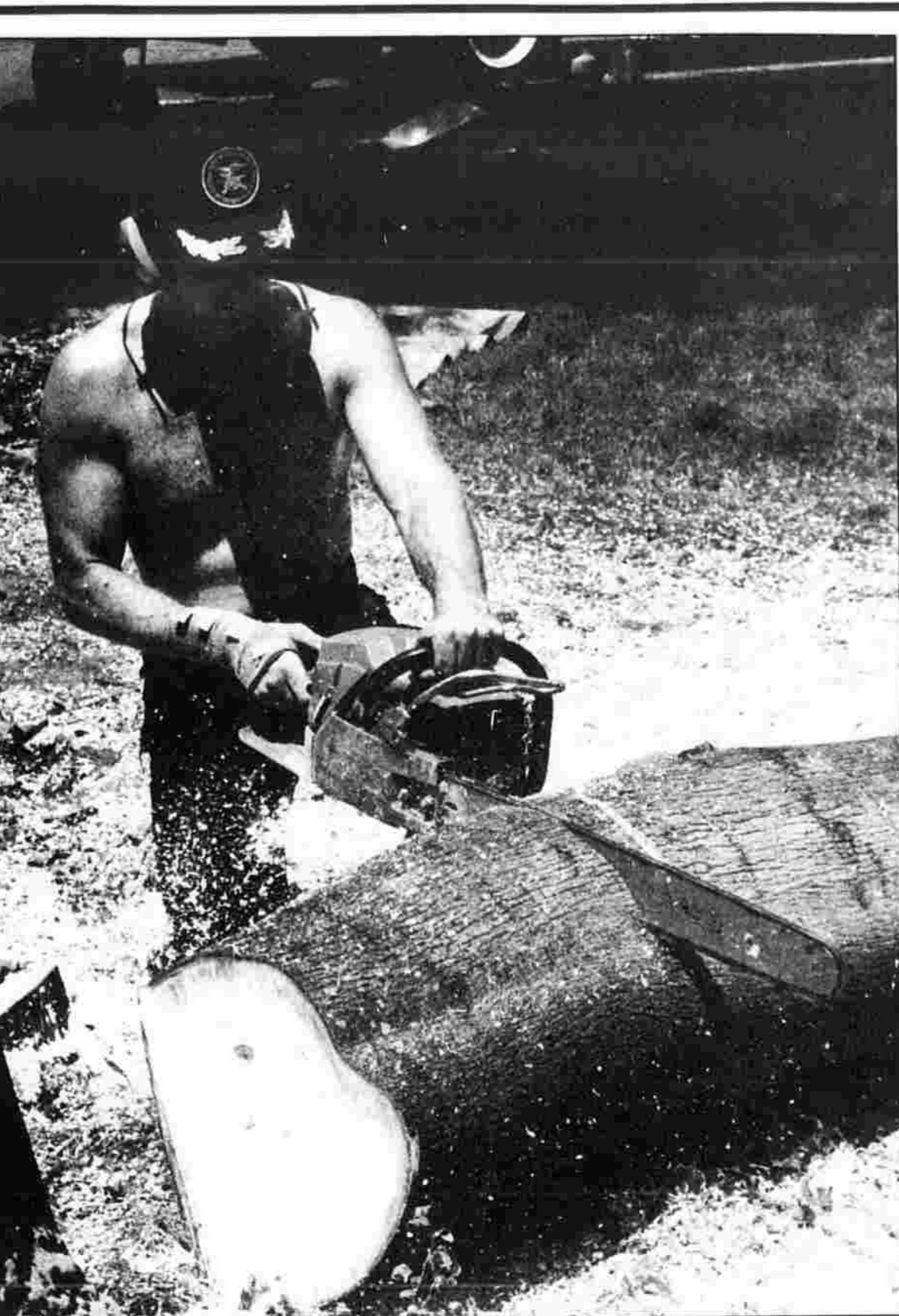
SAWING LOGS — Hans Olsen of Manchester, owner of Olsen Tree Experts, East Hartford, saws a Norway Maple into movable logs. The tree is being removed from 494 Center St. to make way for a stone wall.
